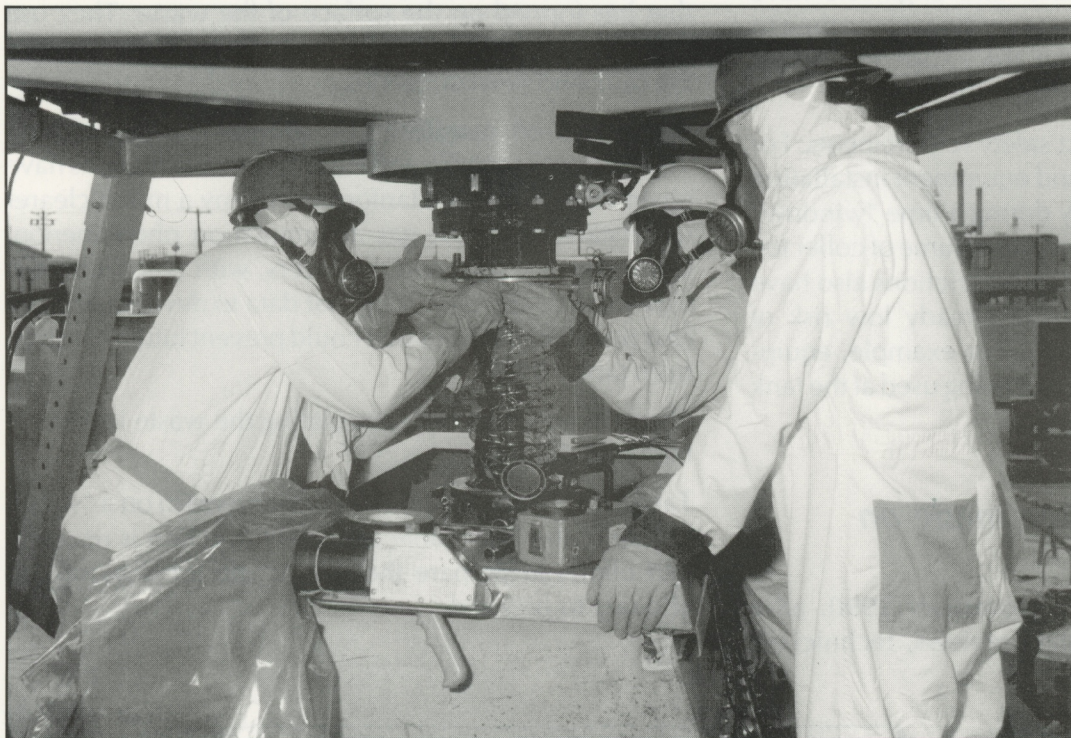
Hanford workers connecting containment bellows at tank 101-SY during the "safe window" after a tank venting.
