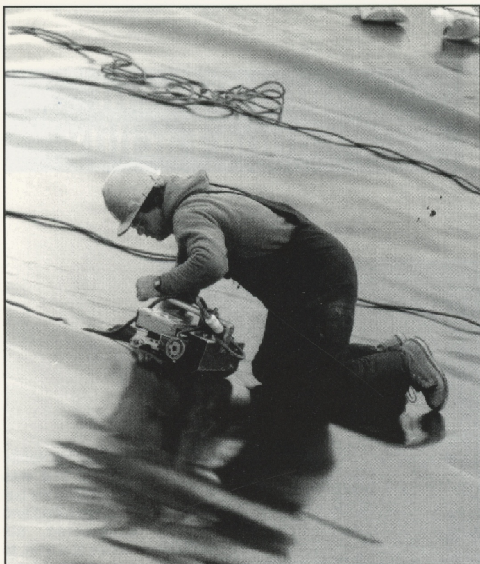
LERF construction began in the spring of 1990 and is due to be completed prior to the restart of the 242-A Evaporator.
